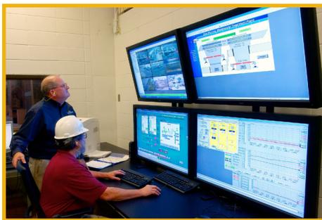
Van Meter brought in ECT, a Rockwell Automation® Process System Integrator. ECT performed a site survey to determine the potential energy savings and increased functionality that could be achieved with a new ECT-supplied blower control system. ECT demonstrated that it could operate the blowers at a lower flow rate that would provide energy savings and still meet DO and minimum mixing requirements.
